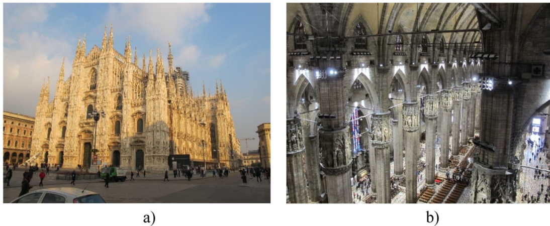
Fig. 3.1. Milan Cathedral: (a) South-West view of Milan Cathedral, (b) Iron tie rods inside the church.
